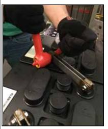
FIGURE 1.4.7 - Torquing connections
