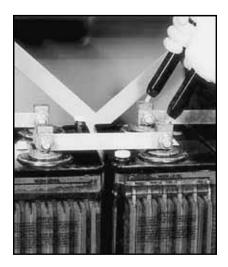
FIGURE 4.2.10 - Measuring internal cell ohmic values
